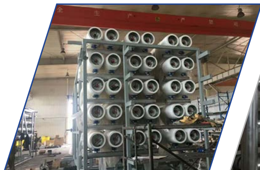
Daya Bay Cnooc's refinery project. July 2016
