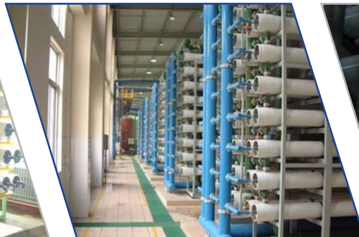
Biel Crystal water treatment engineering. May 2015
