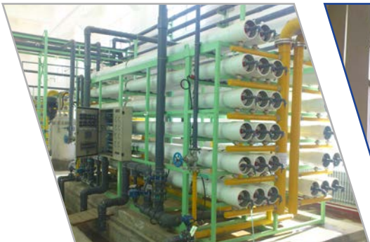
Gansu chemical plant water process engineering. May 2014
