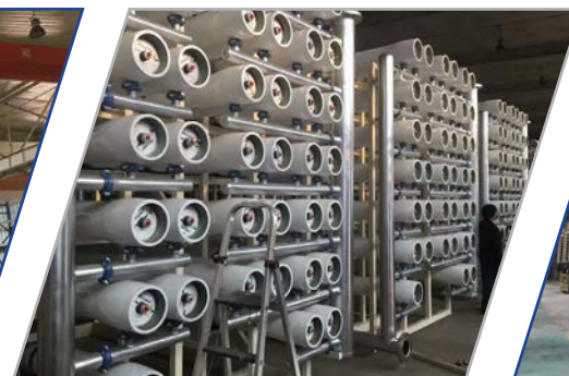
Qingdao wastewater reclamation project. Aug 2016
