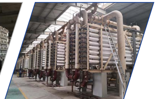
Dalian Hengli petrochemical water treatment project. Nov 2017
